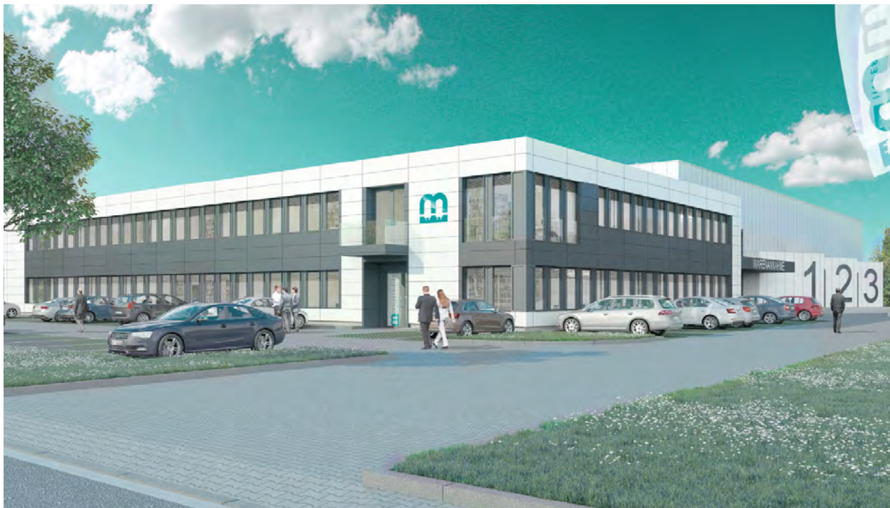
The MULTI-LITE building in Reinbek
