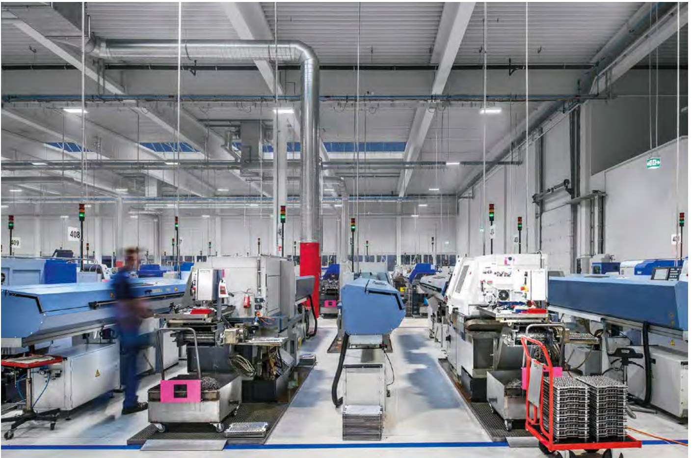
↑ Diesel SpA, Molvena | IT Architektur: Diesel Creative, Breganze / F & M Ingegneria SpA, Mailand | IT Lichtlösung: CRAFT, ECOOS, IYON
